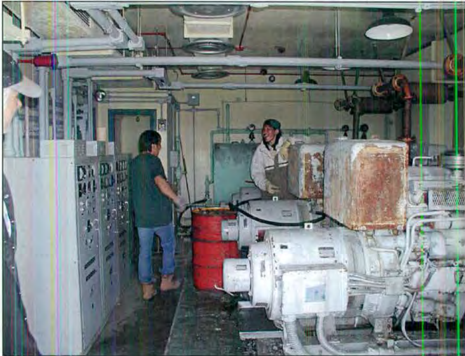
Photo 4. Draining the generators at site 309 (10 June 2001).
