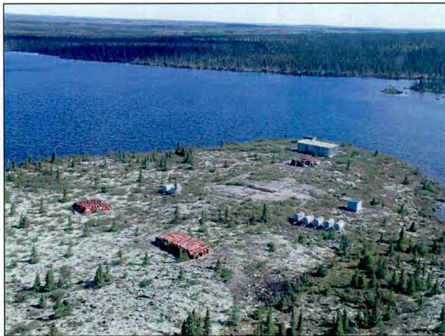
Photo 16. Aerial view of site 315A following completion of clean-up work (8 June 2001).
