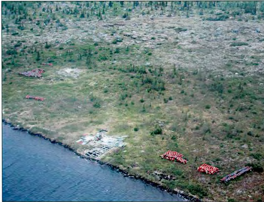
Photo 2. Aerial view of site 224A following completion of clean-up work (14 June 2001).
