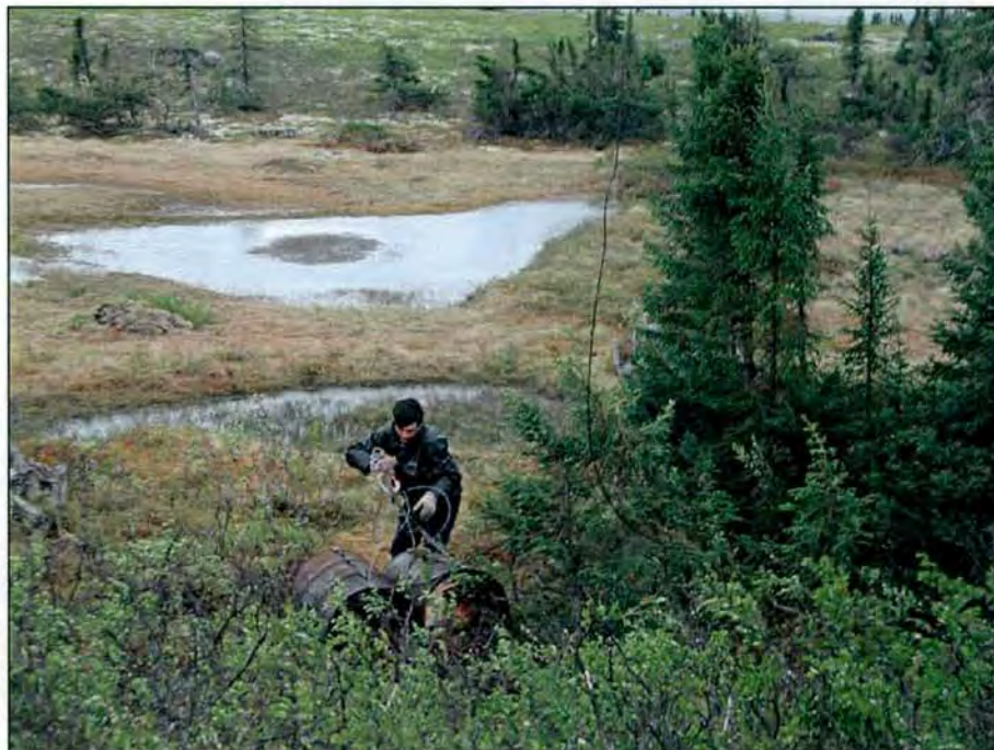
Photo 13. Utilization of a sling to remove two barrels containing hydrocarbons from site 315 (4 June 2001). Note the proximity of the wetland.
